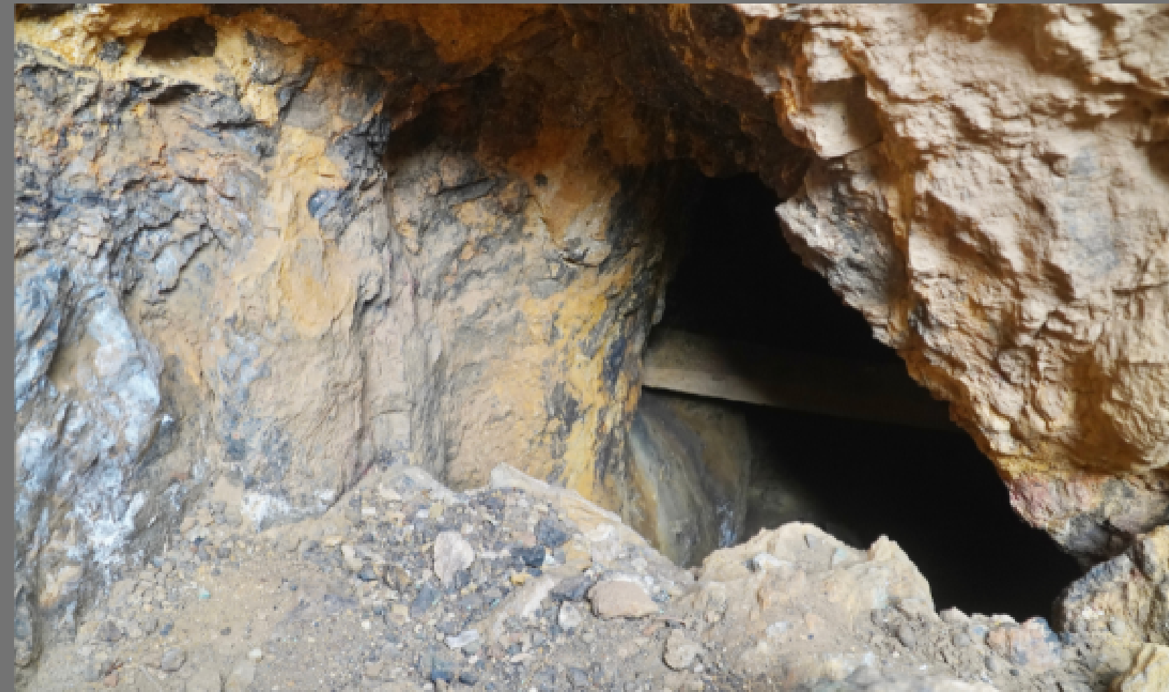
WOODEN SUPPORT IN ADIT
