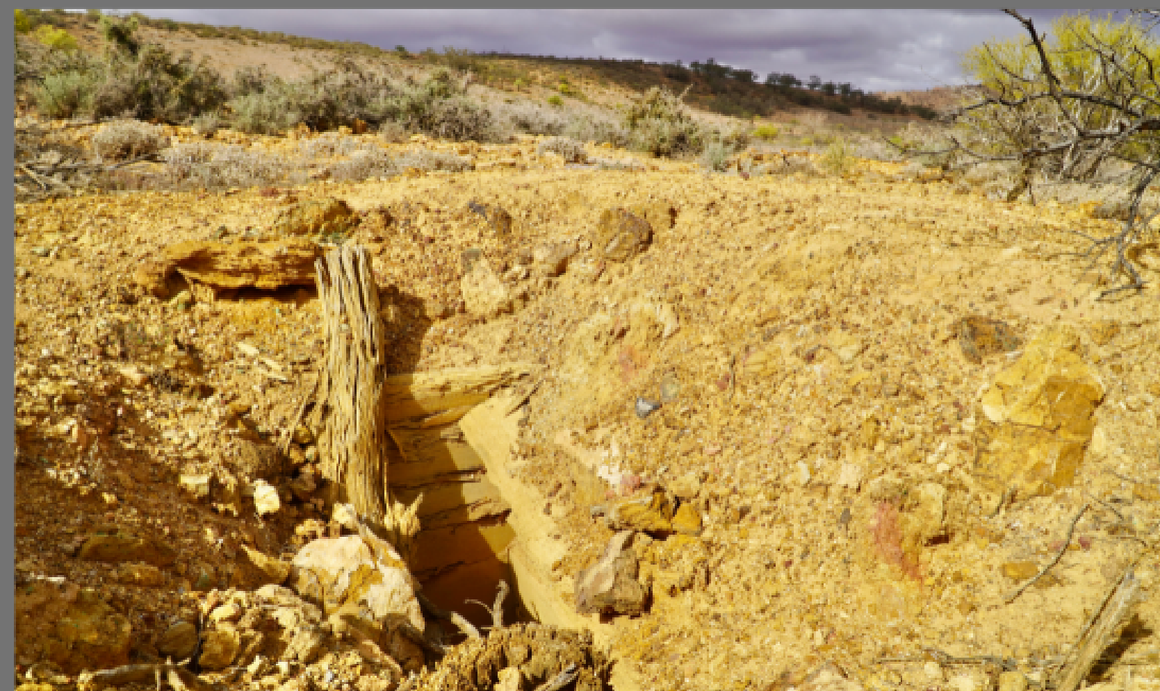
WOOD TIMBERING IN VENTILATION SHAFT (1/3)
