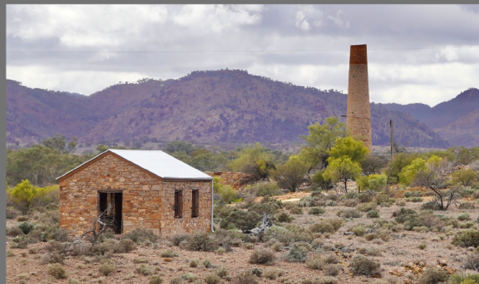
RESTORED ROOF OF THE ASSAY OFFICE
